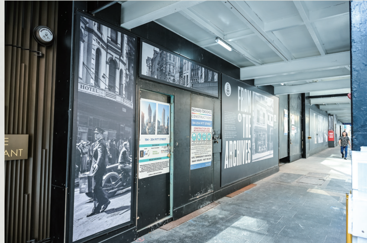
Photo 7: Construction site fencing in Sydney’s historic district.
