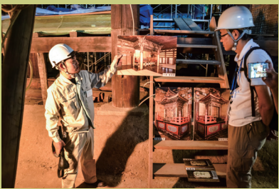
Photo 3: Restoration site of the Main Hall of Honryu-ji Temple, Kyoto. Pre- and post-restoration photographs were displayed at key points around the site to help visitors clearly understand the differences before and after restoration.
