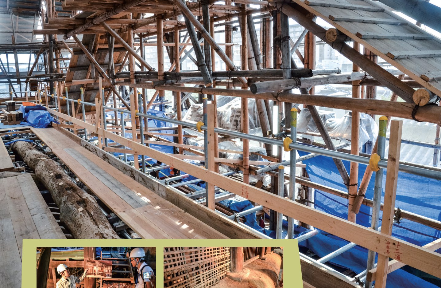
Photo 2: Restoration site of the Main Hall of Honryu-ji Temple, Kyoto. Safe pathways were installed along the construction scaffolding to enable visitor access.
