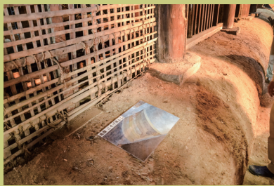
Photo 4: Restoration site of the Main Hall of Honryu-ji Temple, Kyoto. After the complete removal of the surface plaster layers of the kamebara, explanatory photos were placed on the exposed surface to illustrate the stratification discovered during dismantling.
