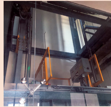
Picture 5: The newly installed elevator in the Museum in 2020 required the removal of the existing floor, which does not align with the concept of reversibility. However, this decision was driven by a desire to achieve universal cultural accessibility and promote the values of cultural equality.
